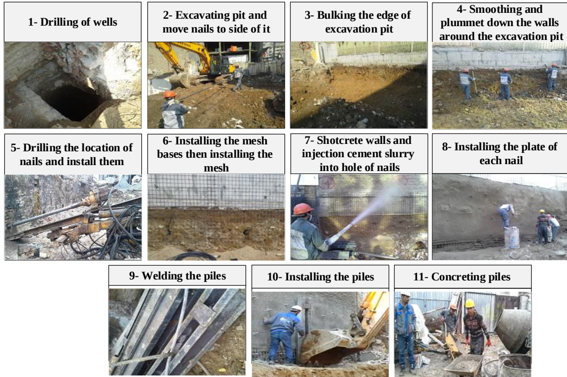
Figure 3. Different activities done in each round of excavation and stabilization operation
